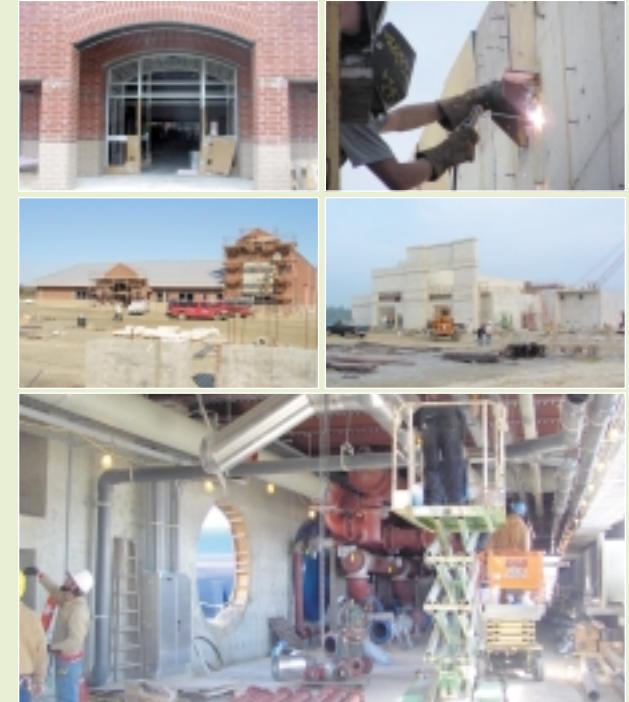
LAKE GASTON WATER TREATMENT PLANT CONSTRUCTION.
