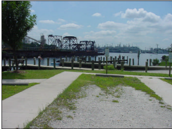
The Jordan Bridge
